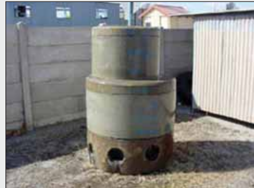
Complete Manhole with access Shaft
