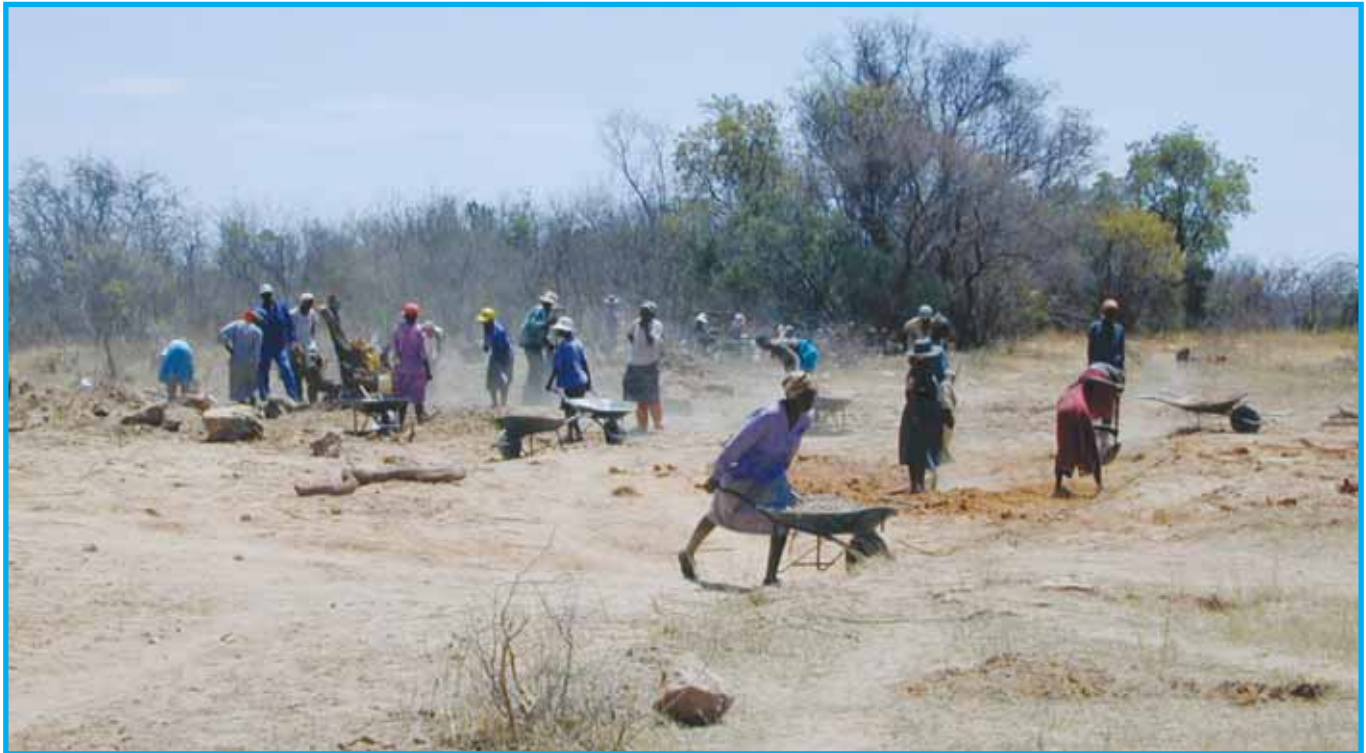
Figure 7-1: Site Clearing by Employment Intensive Construction
