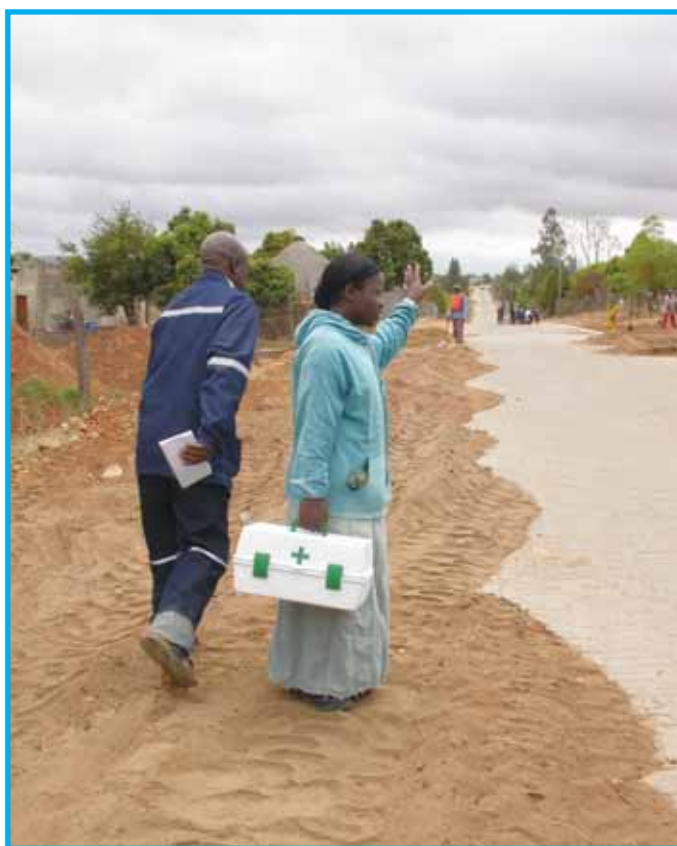
Figure 10-2: First Aid Officer on site
