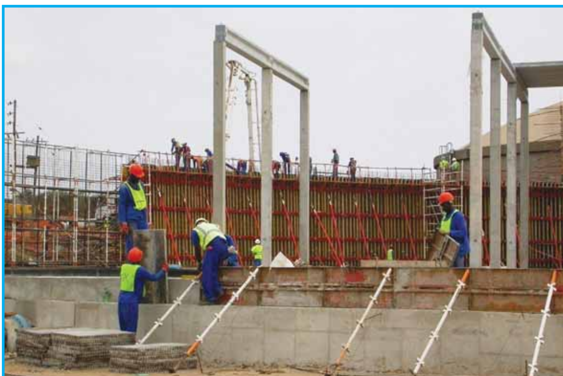
Figure 3-8: A Reinforced Concrete Reservoir under construction in Polokwane, SA
