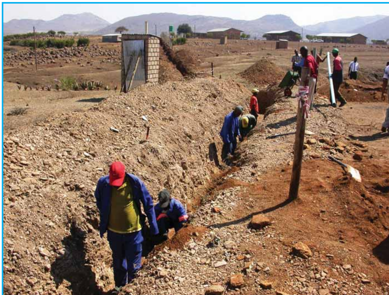
Figure 2-1: Trenching for water pipe installation
