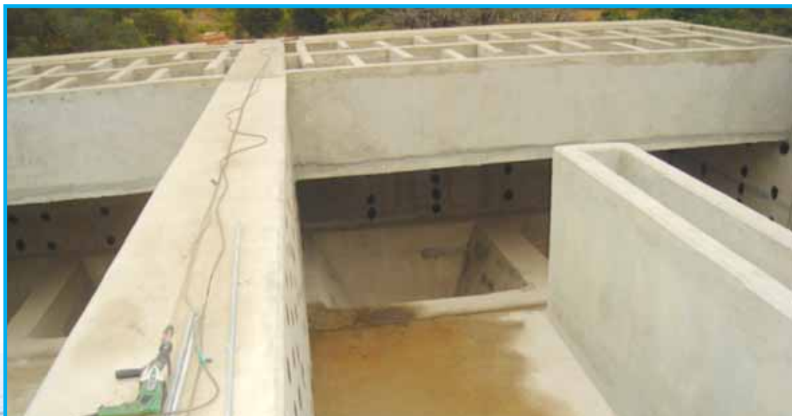
Figure 3-6: Construction of a Clarifier in Vhembe District, RSA
