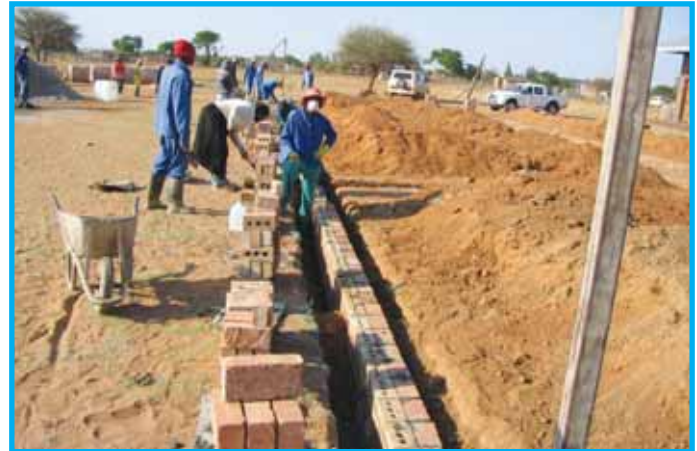
Figure 9-1: Brick work in a construction site
