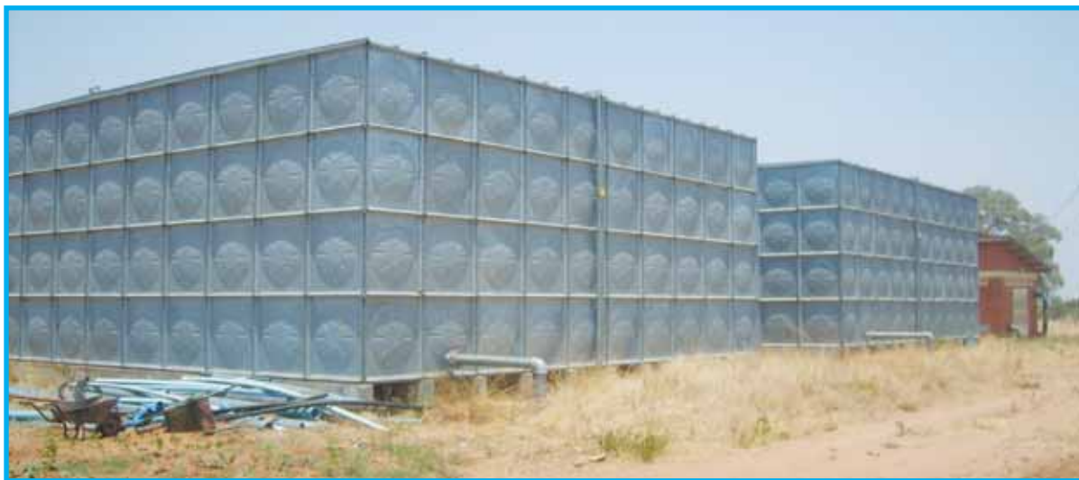
Figure 3-7: Sectional Steel Ground Reservoirs in North East District, Botswana
