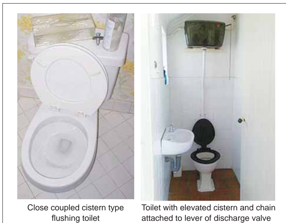
Figure 4-10: Commonly used Water Closets
