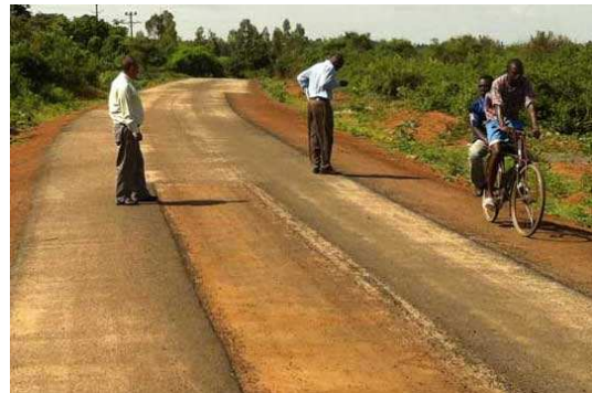
Surfacing works in Bondo
