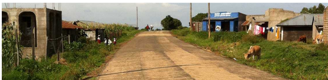
Completed road section in Bondo
