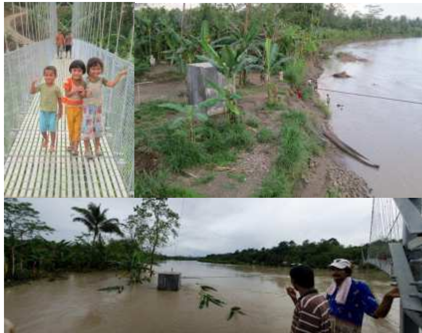
Fig 4(a) Oyo River bridge (b) wind guy anchor block near the eroded river bank (c) flood of the 11-12 November, 2012, inundating the river bank including the wind guy anchor block.
