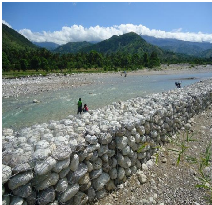
Photo 3. Gabion Wall in Port-à-Piment
