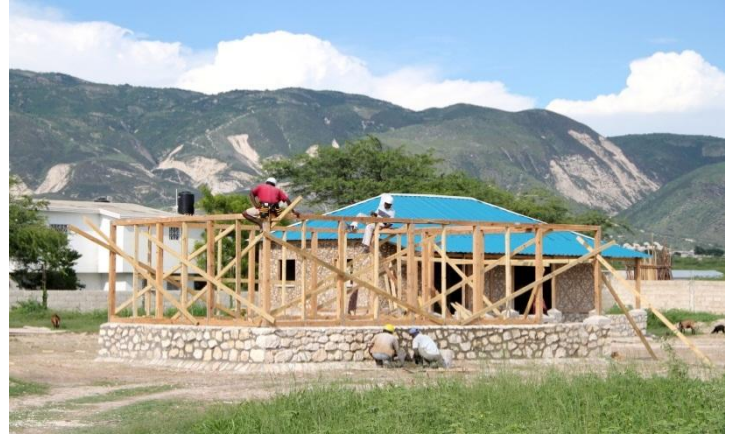
Photo 2. Building housing: over 20 per cent of the debris has been recycled and used in various low-cost, earthquake-proof, cyclone-proof building works in harmony with Haitian architecture (© UNDP/M. Solon).
