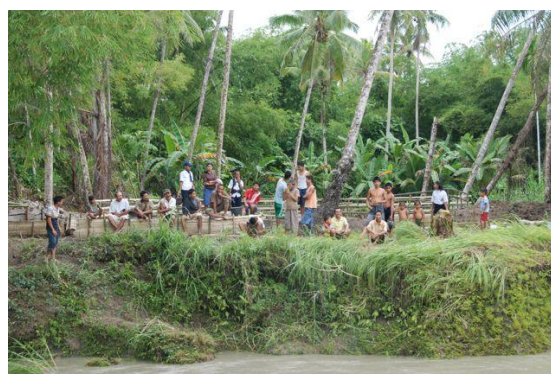
Figure 10: community preparing bridge foundation
