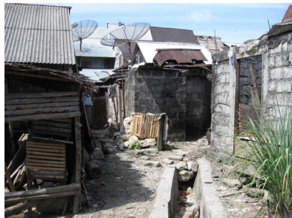
Figure 16: open sewage discharge
