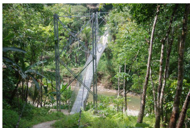
Figure 7: Modular Suspension Bridge
