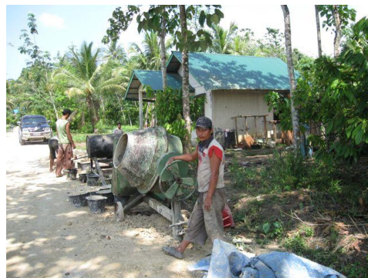
Figure 3: mixing pavement materials
