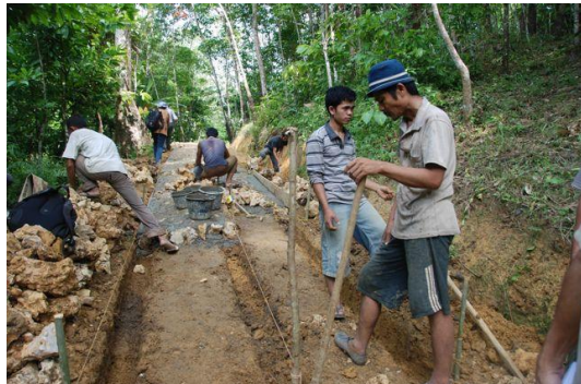
Figure 9: contractor at work
