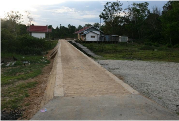
Jetty approach in Lawang Kajang
