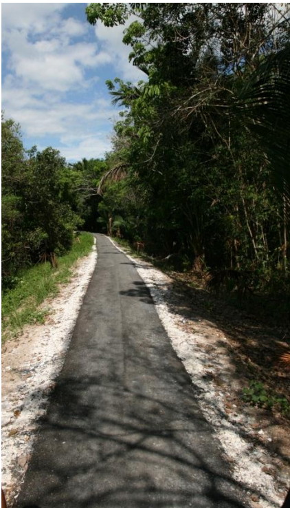
Cold mix path in Pilang
