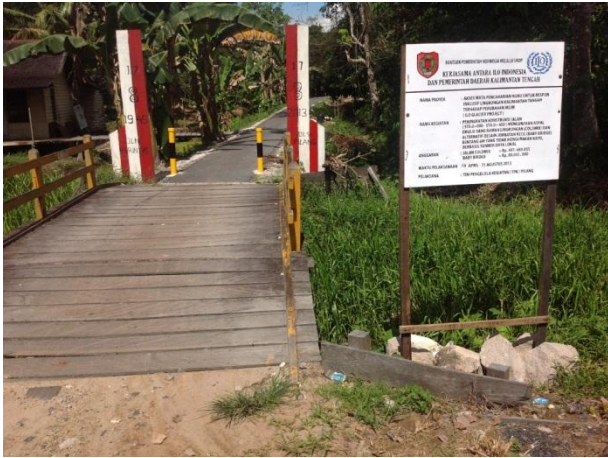
Cold mix path (400m) in Pilang
