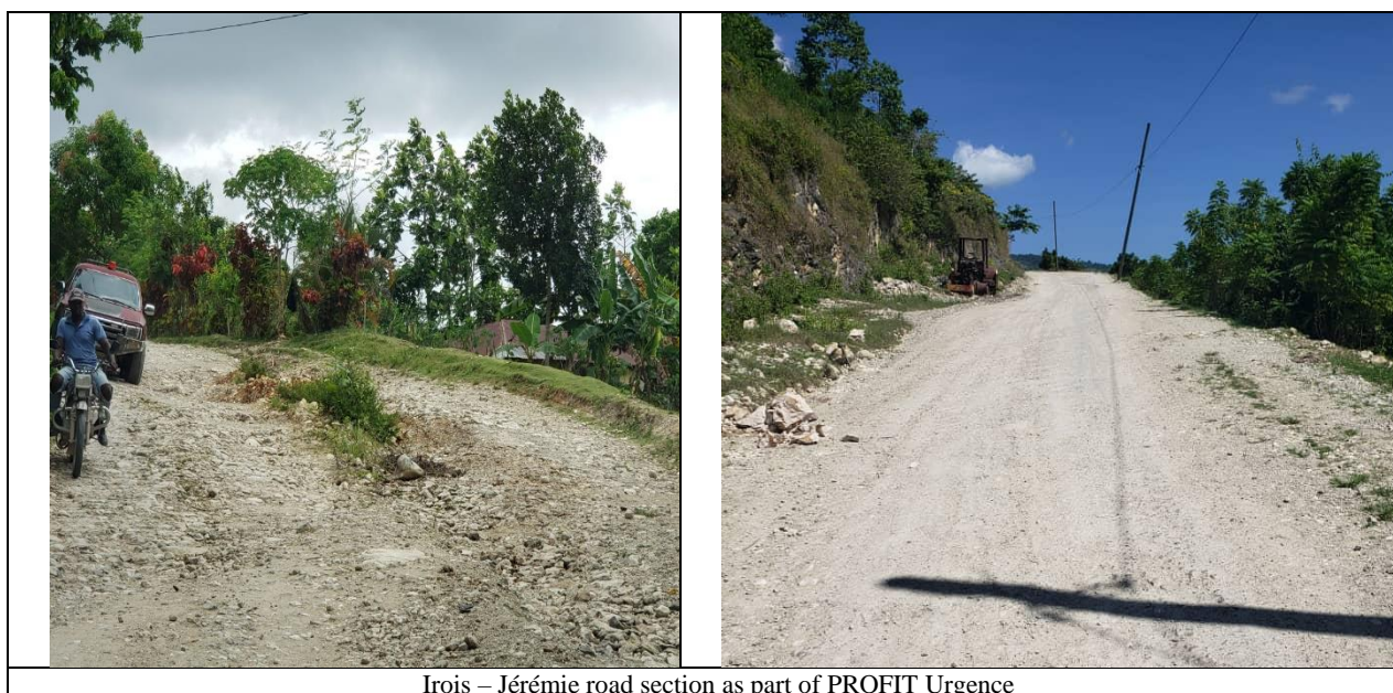
Irois – Jérémie road section as part of PROFIT Urgence
