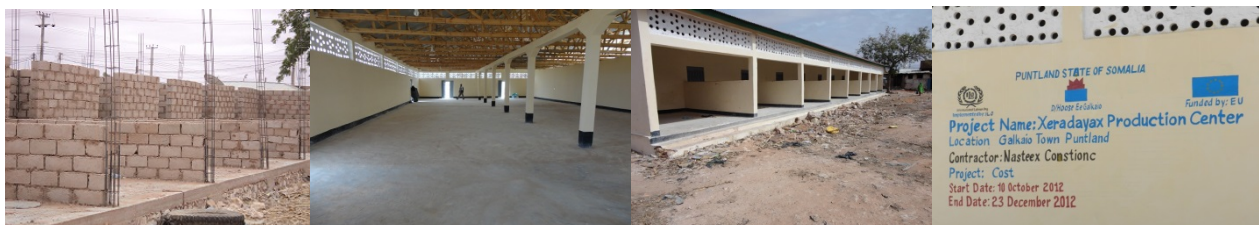
Source; technical progress reports and photos taken during evaluation mission
