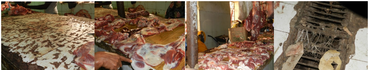
Photo set 6: Worn-out services, use of cartons and loose drainage cover that poses risks of injury
