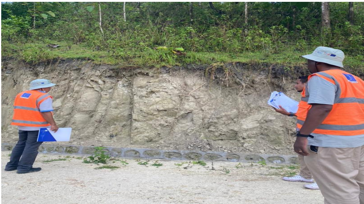
March 14, 2022 visual site inspection of Souru-Nairete Road, Lautem Municipality. Gravel road section, lined side drain.
