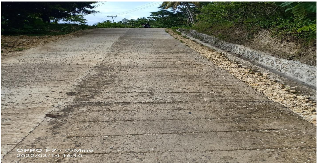
March 14, 2022 Visual site inspection of Souru-Luturula Road, Lautem Municipality. Overall, the plum concrete section is in good condition.
