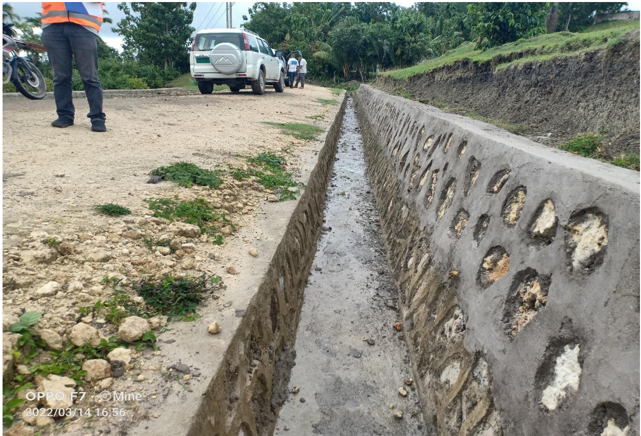
March 14, 2022 visual site inspection of Souru-Nairete Road, Lautem Municipality. Gravel road section, lined side drain.
