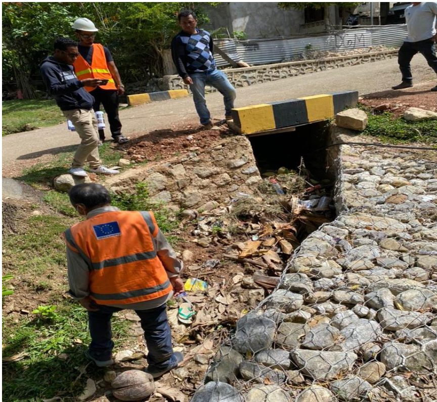
March 15, 2022 visual site inspection of Apatmutu-Larimi-Canfuro, Lautem Municipality. During the rainy season cross-drains such as this need frequent clearing as part of routine maintenance.
