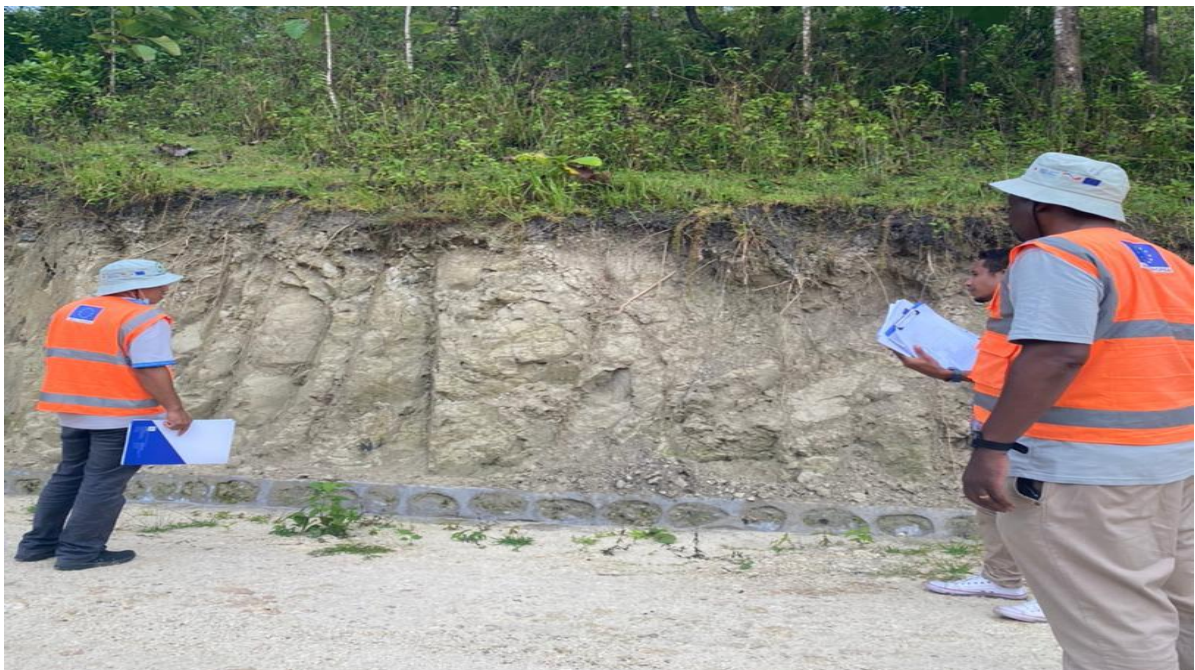
March 14, 2022 visual site inspection of Souru-Luturula road, Lautem Municipality. A section with risk of landslide. Construction of retaining wall needed?
