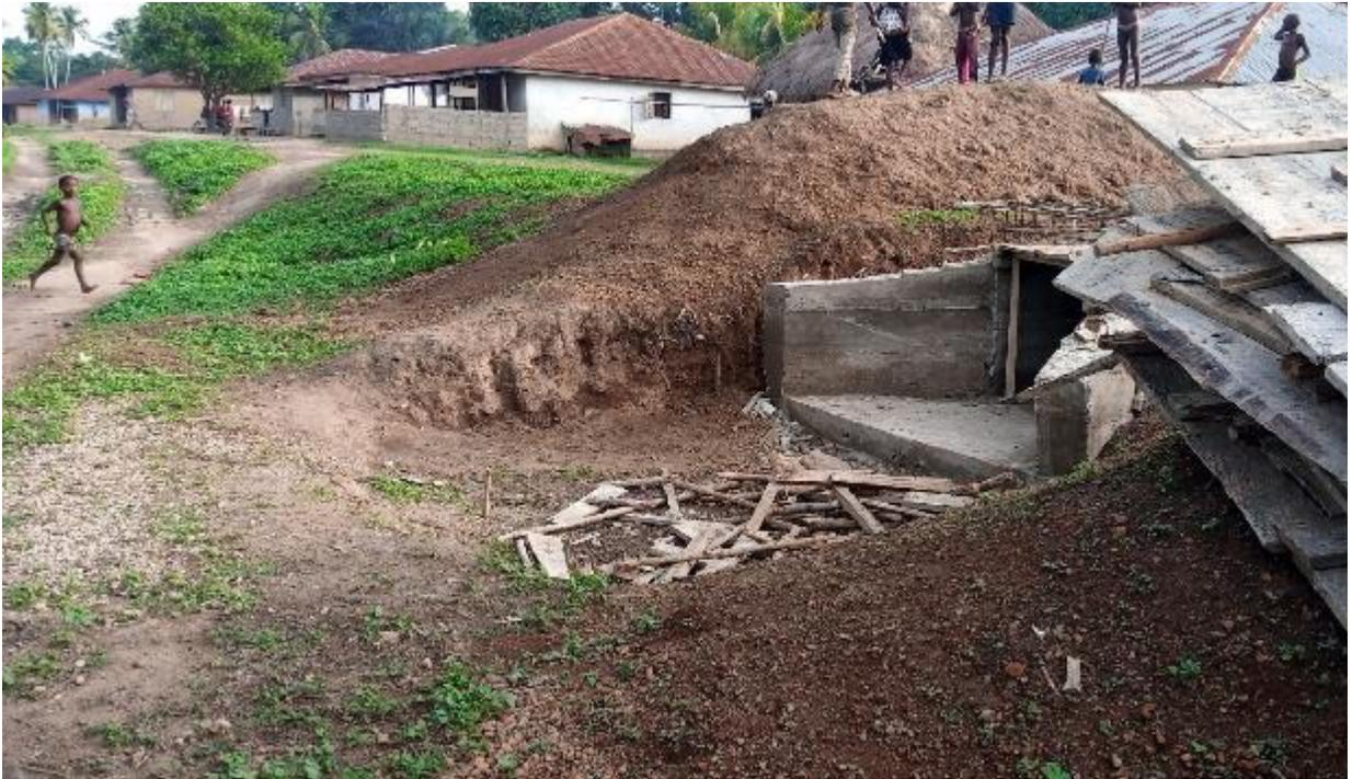
*Photo 3: A Culvert Under Construction*
