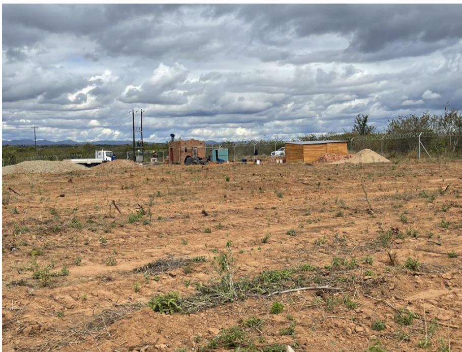
Picture 2: Construction works at the Mercury Free Gold Milling Plan
