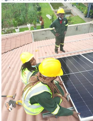
Figure 4 Beneficiaries installing solar PVC
