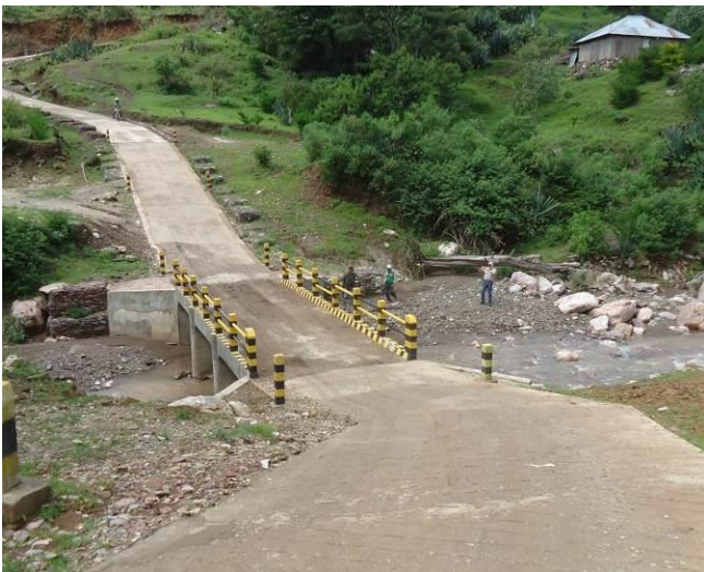
The much safer upgraded stream crossing near Falubosa.
