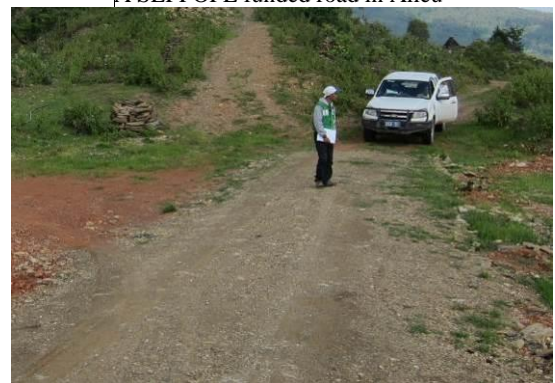
Joining onto the ERA rehabilitated road
