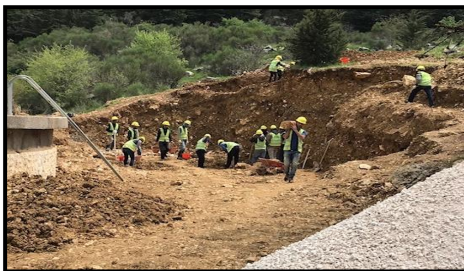
Photo 1 - EIIP Workers in Akkar, Tal Abbas
