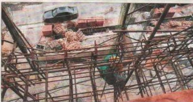
**CARELESS:** While poorly built scaffolds — such as those missing the guard rails required to keep workers from falling — are a key problem, there are also workers who do not attach their harnesses to the struts, a requirement for anyone working above a height of 2m.
