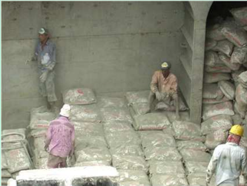
WORKERS UNLOADING CEMENT IN SHIP'S HOLD.
